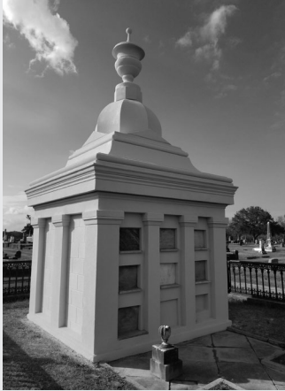
L. M. Wilson Mausoleum after restoration.
