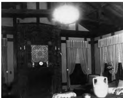
Coca-Cola bottler Walter Bellingrath had Rogers enlarge his fishing lodge in the early 1920's. Here is a view of the living room, ca. 1930. That building was demolished in 1962 but elements of the interior design are reflected in the interior of the nearby Chapel completed in 1939.
