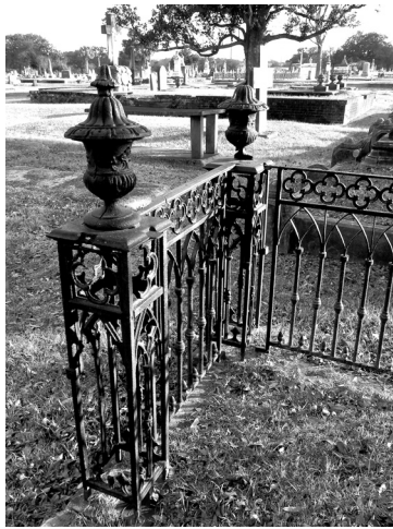
A handsome gothic cast iron fence once surrounded the Dunn lot. Here a corner survives.
